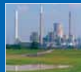
Orion Power Dhaka Ltd.
