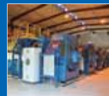
Digital Power & Associates Ltd.
