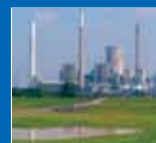
Orion Power Dhaka Ltd.
